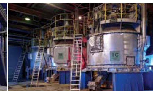
Power Station equipped with LOESCHE classifiers - Ratcliff, UK
